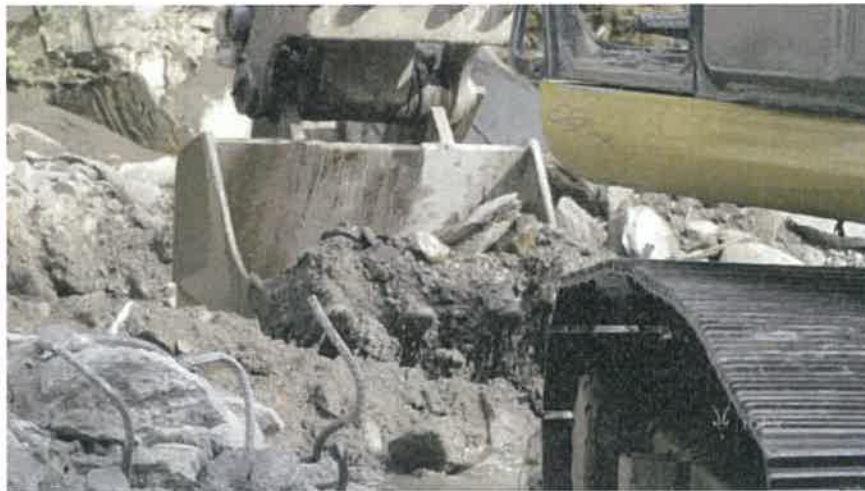
Geer Dam Removal 8/17/17
