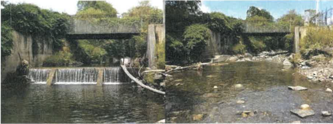
Before (left) and after (right) photos of the Geer Dam Removal.
