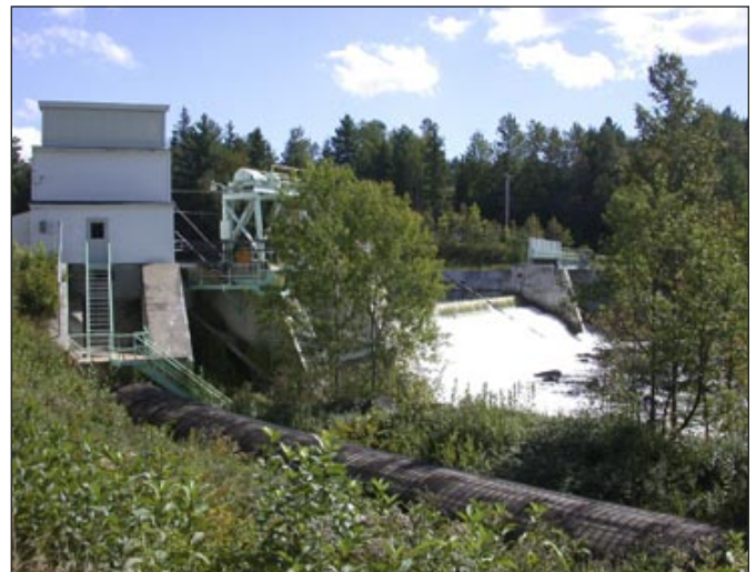
Canaan Dam and its historic wood stave penstock between Canaan and Stewartstown, a few miles from the Canadian border. The dam is up for relicensing.
