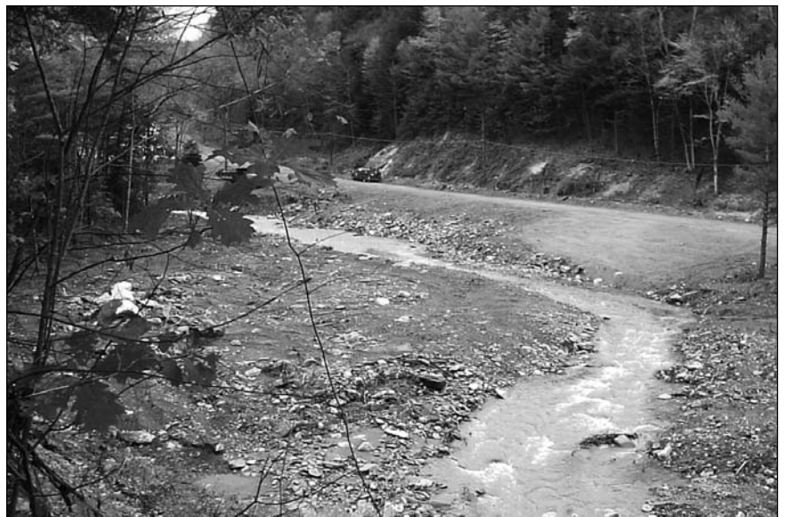
AFTER THE FLOOD —Warren Brook, formerly a bucolic woodland stream, is completely transformed by flooding last fall. This photo from the N.H. Department of Environmental Services shows gravel and glacial till exposed in the brook's washed out banks.
