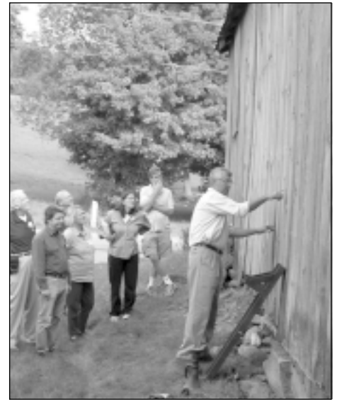
Stephen Bedard of Henry Page House Restoration in Gilmanton, NH, draws attention to early hand-made nails used in barn siding.
